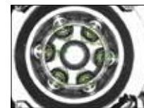
Drive Shaft Inspection
